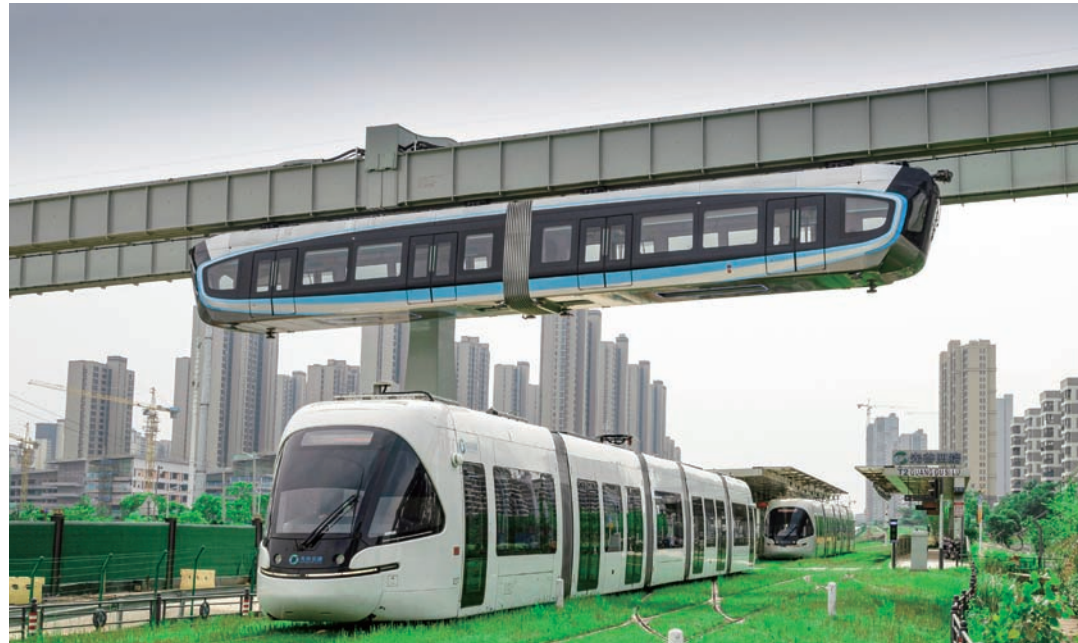
“光谷光子号”空轨和“光谷量子号”有轨电车（叶茂青 摄） “Photon” Air Rail and “Quantum” Tram in Optics Valley (photo by Ye Maoqing)
